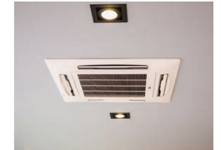
Upgrading production/air-conditioning equipment to high-efficiency models
