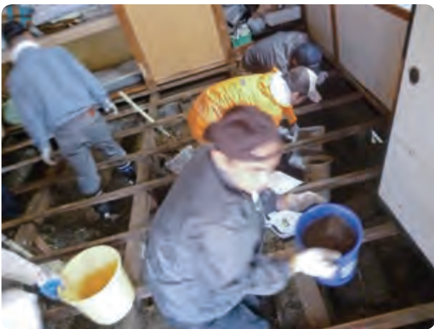
Helping to move households and remove mud from flooded homes
