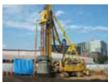
Ground pollutant cleanup
