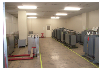
PCB Storage Shed at Victor Creative Media
