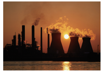
Power plant where ATEX radios are used
