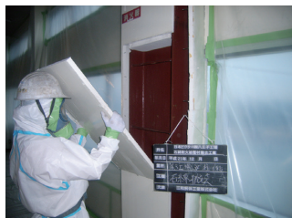
Asbestos Removal Work
