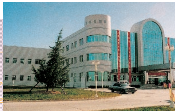
In November 1997, JVC Beijing Electronic Industries Co., Ltd. in China completed a new factory for VCRs and camcorders.
