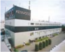
Head Office / Hachioji Business Center
