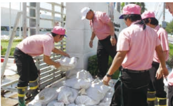
Training at a production base in Thailand: Sandbagging based on flood experience
