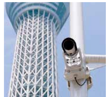
Security camera systems
