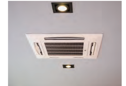
Upgrading production/air-conditioning equipment to high-efficiency models
