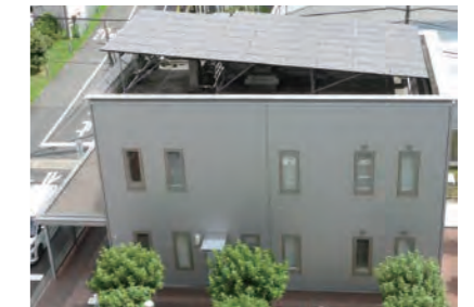
Installation of energy-saving equipment (solar power generation)
